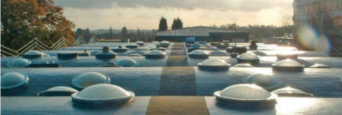
Liquid roofing systems protect the roof structure through a liquid applied solution, which solidifies into a totally seamless, waterproof barrier. The system can be applied to all common substrates and does not require the removal of any existing roofing material. Any failed material such as blisters can be simply cut out, filled and then overcoated. This avoids any need for temporary roofing and keeps contract time to a minimum.
